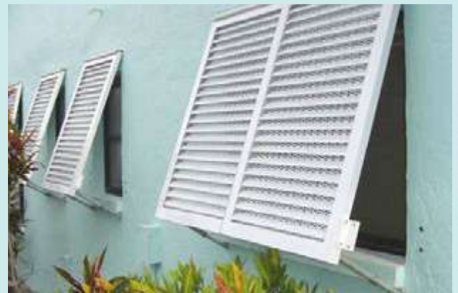
CH5-36: Hurricane shutters remain the most economical solution for most homeowners to protect window openings in a storm, although hurricane resistant glass is increasingly popular.
