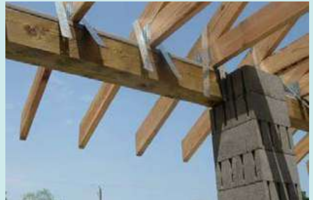
CH5-35: Hurricane straps are able to withstand winds of more than 100 miles per hour. The easiest way to install hurricane straps is during the construction of the home.
