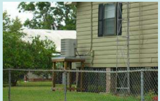
CH5-37: Elevated on a platform above expected flood water, an outdoor condenser unit is securely attached to the platform and will not become damaging flood-borne debris.
