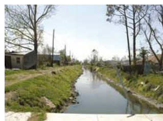
D-28 Drainage way in St. Bernard Parish.
