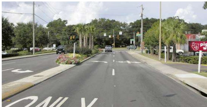
C-13a Existing Conditions
