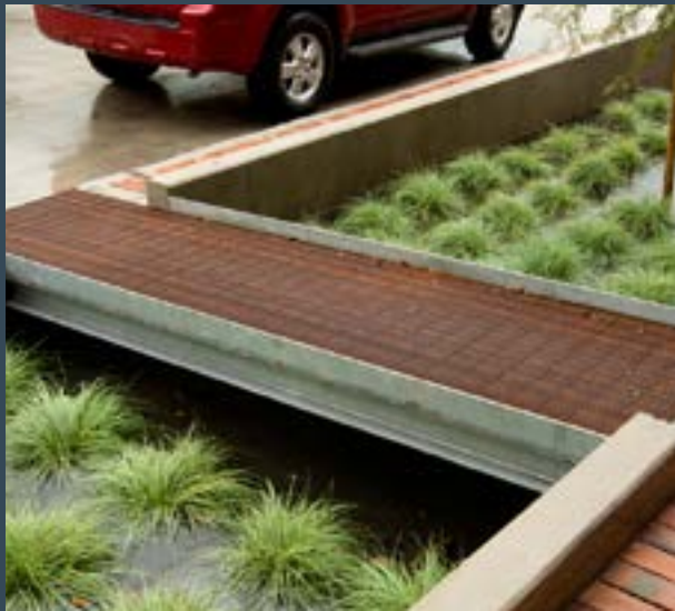
Houston, TX: Curbside rain garden. Example of stormwater management and beautification, part of the Bagby Street Reconstruction project. Image property of Design Workshop.
