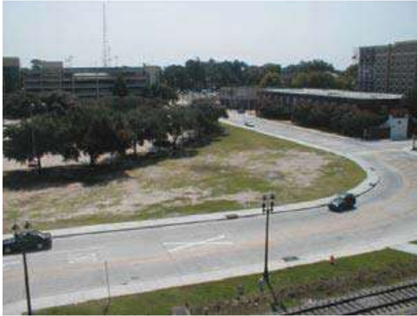
River Road Realignment - Completed May 2002
