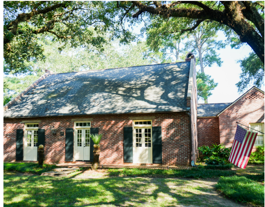
Residential development in Abbeville.
