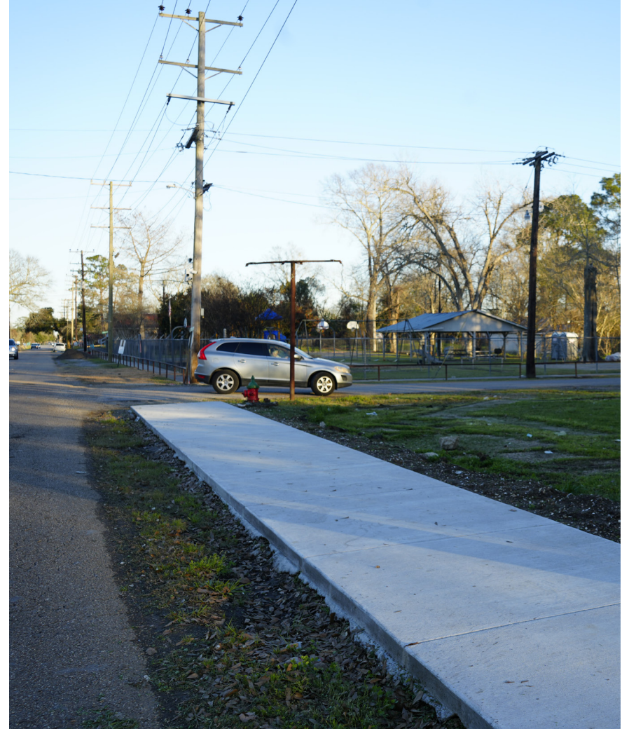
New sidewalk installation along Graceland Avenue.
