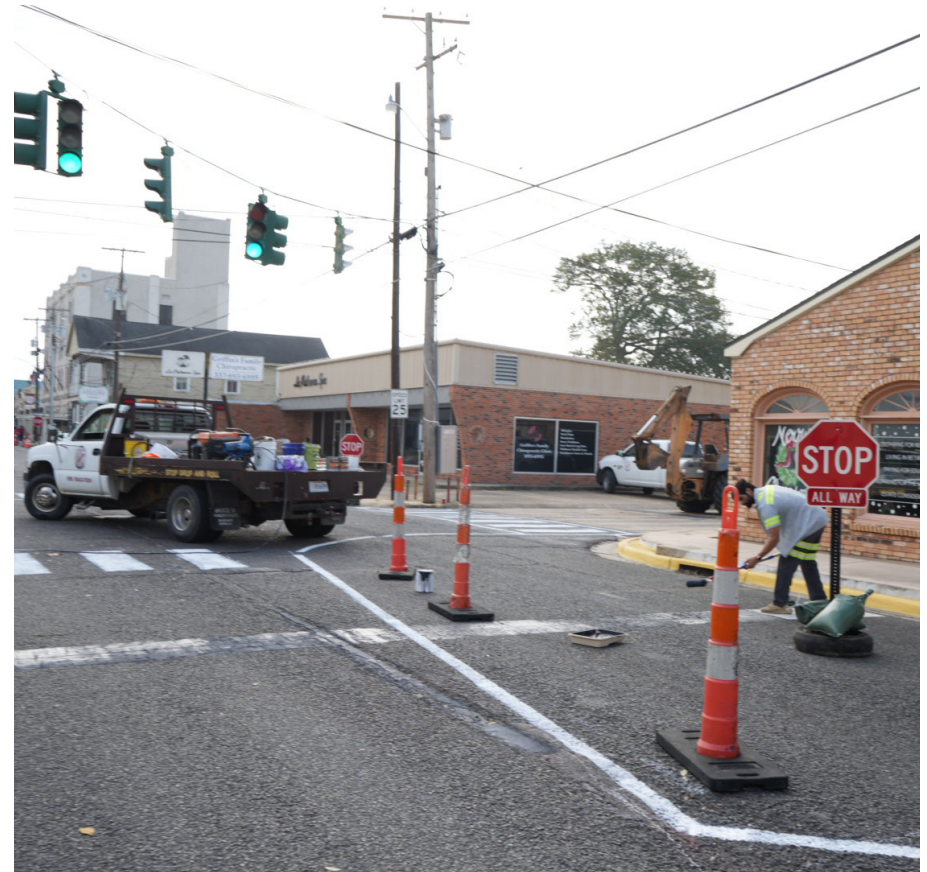
Men working on intersection improvements
