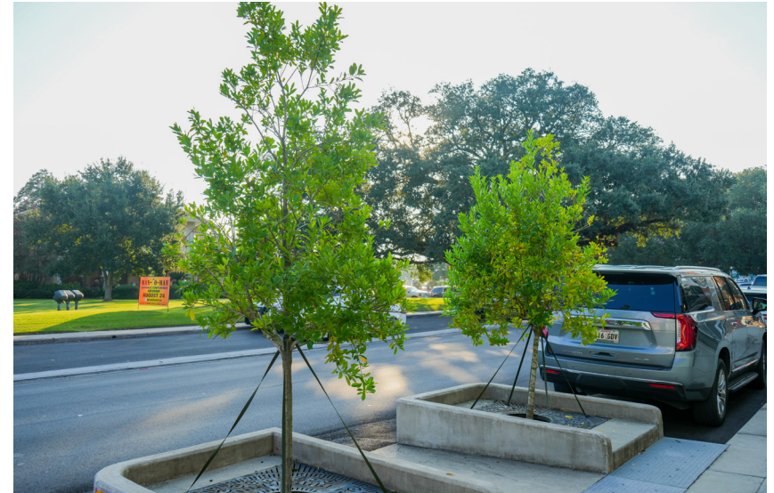
Landscape bulb out planters installed along roadway
