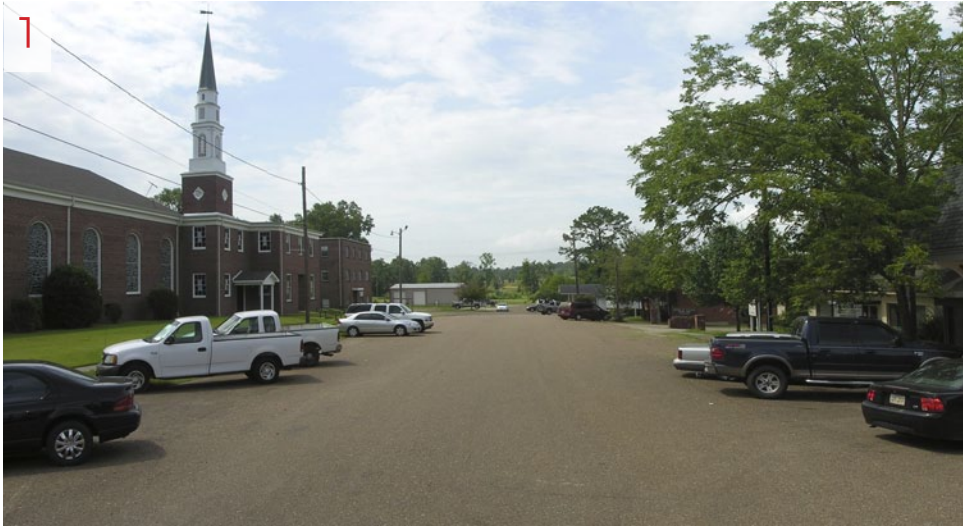
EXISTING CONDITIONS. Looking south down Third Street. The First Baptist Church is on the left.
