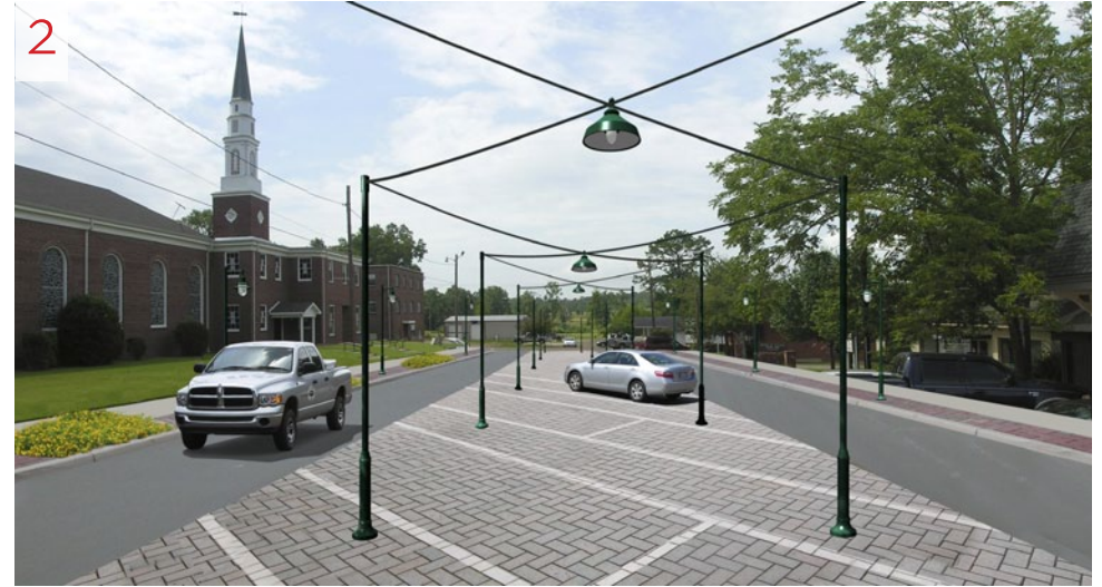
Sidewalk on both sides of the street improved. Angled parking with pervious pavement added to the center of the street. Lighting installed that hangs from overhead wires.
