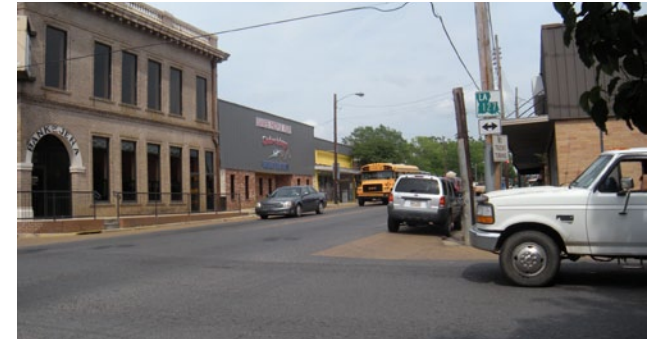
Truck-turning movements between Highway 84 and LA 127 require considerable attention with respect to roadway planning and design.
